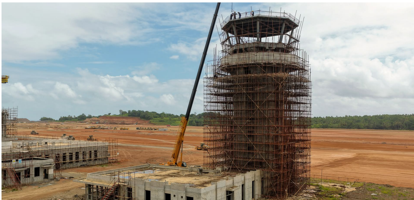
The Dominica International Airport under construction, a flagship investment project underpinning the Commonwealth of Dominica's economic transformation.
