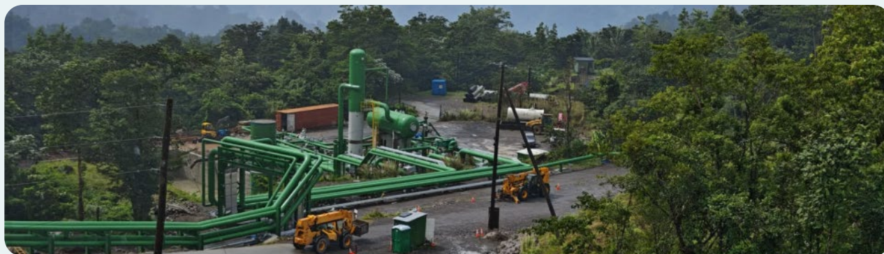
Dominica geothermal plant under construction (source: facebook/ Vinir Dóminíku)
